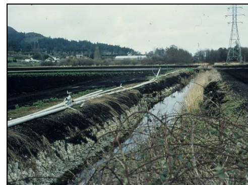
Figure 1: Ditch prior to restoration, early 2000
