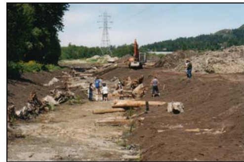
Figure 4: Creek under construction
