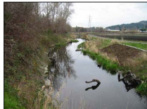
Figure 5: Completed creek late 2002
